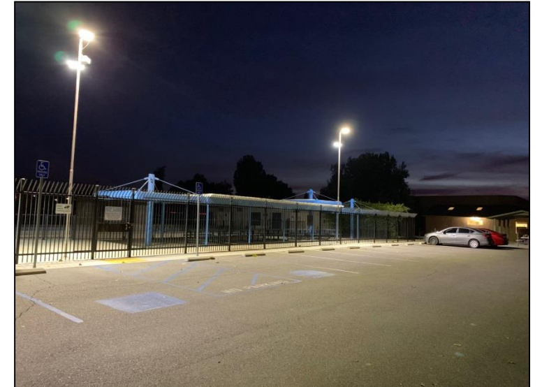
Upgraded Sallee Park lighting to LED
