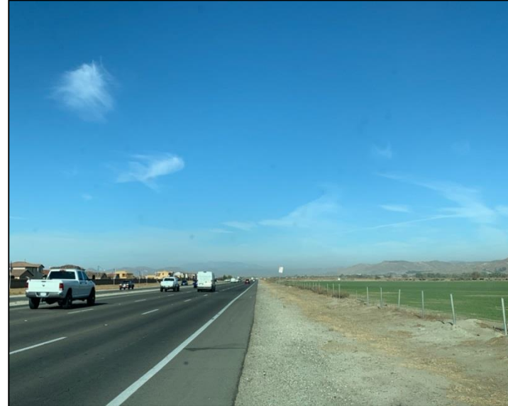
Over 79,000 LF of the City Right of Way was cleaned
