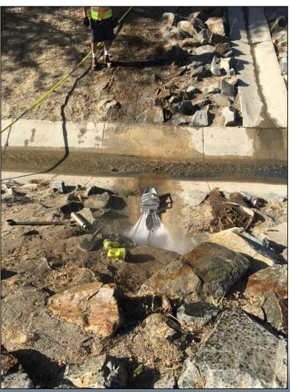
The new Vactor's high powered nozzle and tools have enabled staff to more efficiently jet and vacuum storm culverts & pipelines throughout the City.
