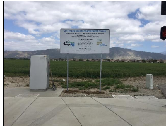
Installed 2 Sanderson Ave Safety Project Signs
