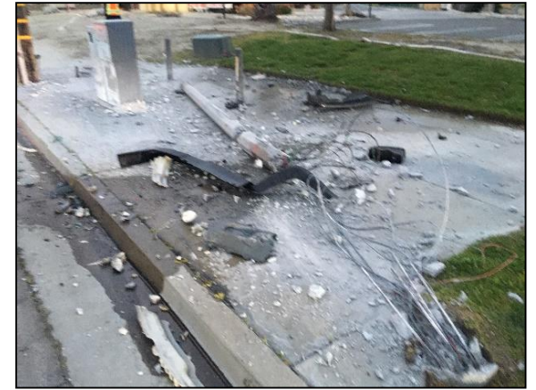
Repaired 2 Streetlight Knock Downs
