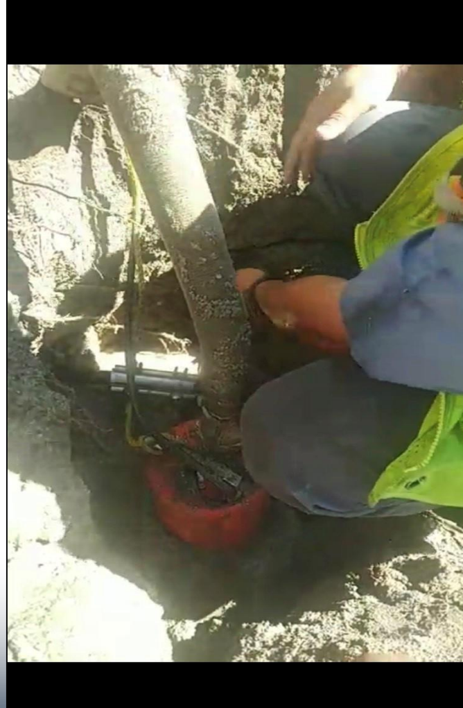
Service Line Repair 272 Maple Court
