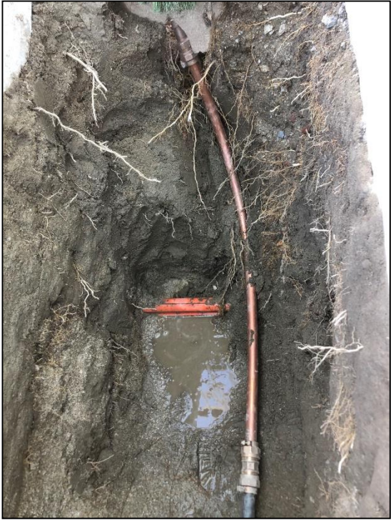
Service Line Leak Repair at 435 Potrero
