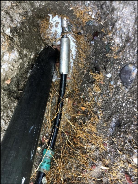
Service Line Leak Repair at 435 Potrero
