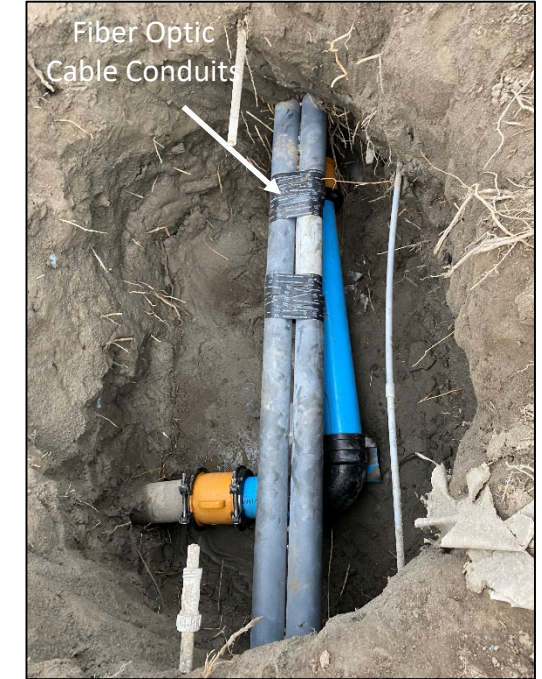
Taco Bell's service line leak under fiber optic cables at Ramona Boulevard and State Street
