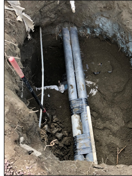
Taco Bell's service line leak under fiber optic cables at Ramona Boulevard and State Street
