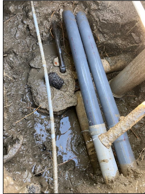
Taco Bell's service line leak under fiber optic cables at Ramona Boulevard and State Street
