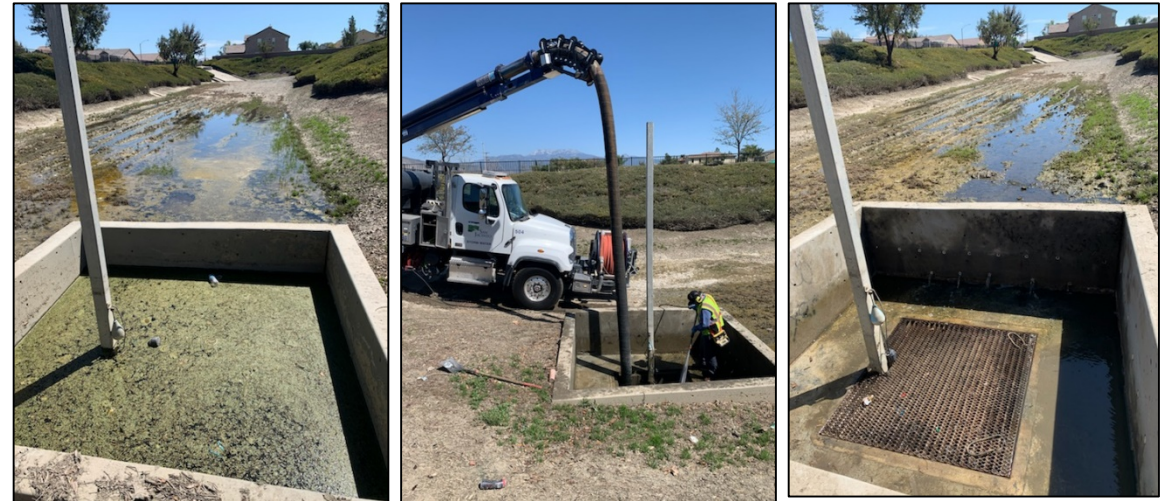
Clearing the storm water basin vault in The Ranch development
