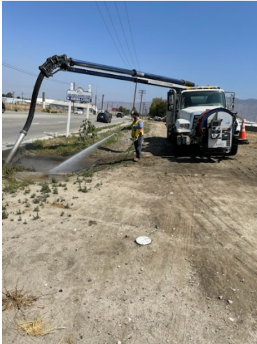
Line clearing on under State Street near Crow's Nest PI
