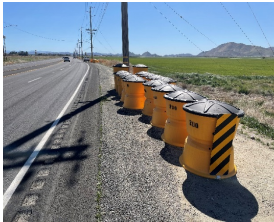
Replaced 12 crash barrels along Sanderson Avenue
