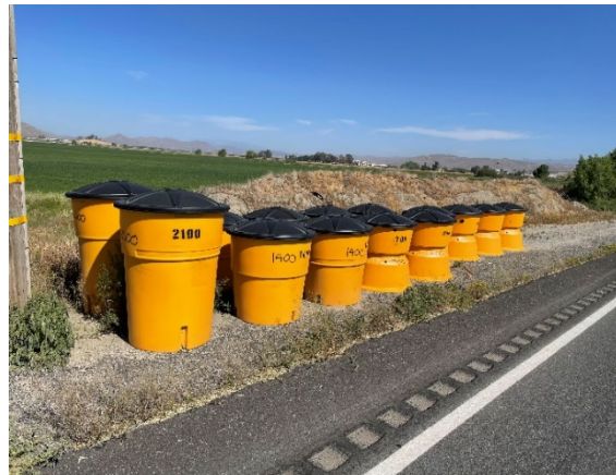
Replaced 12 crash barrels along Sanderson Avenue
