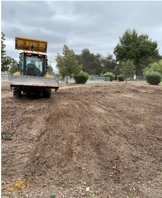
Grading and leveling area for the Community Garden at Sallee Park
