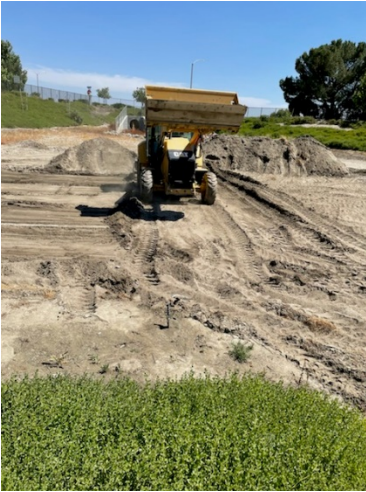
Sand Removal from Luz del Sol basin
