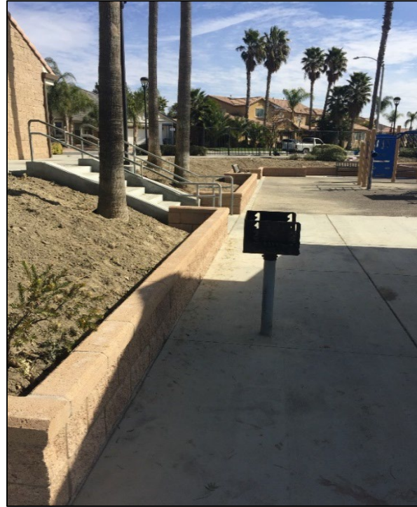
Retaining walls installed at Millett Park
