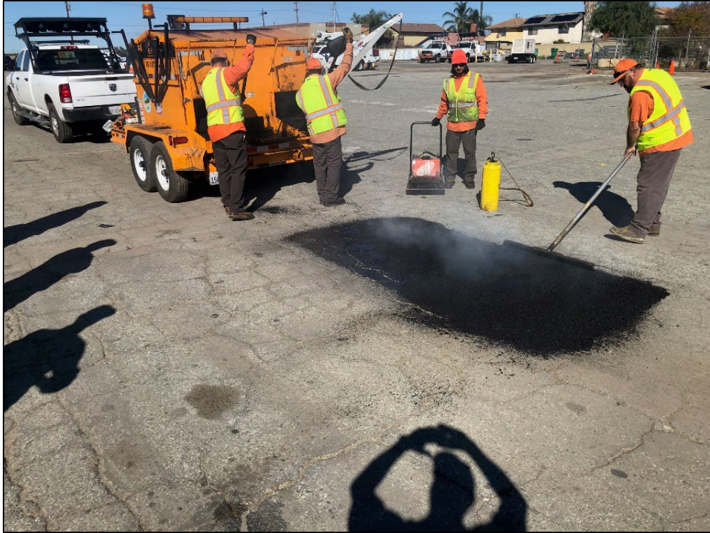
Crew received asphalt hot patch demonstration by CRAFCO
