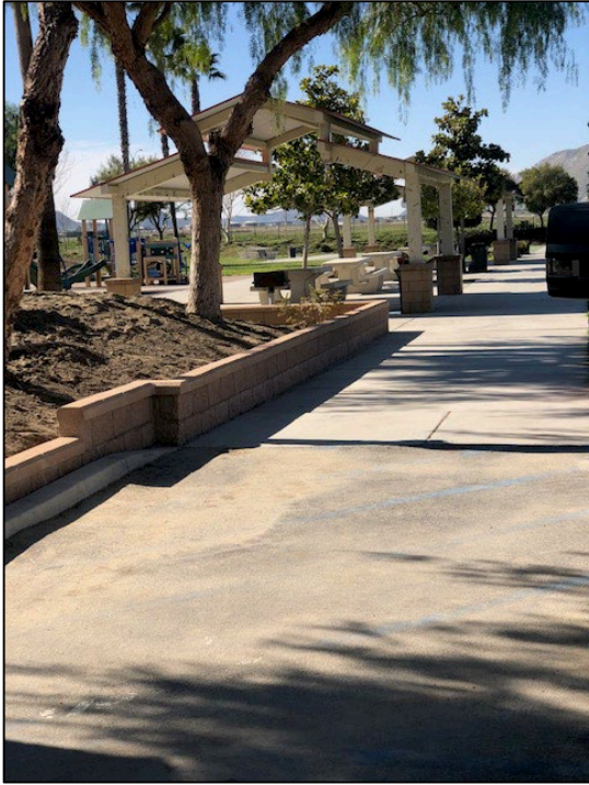
Retaining walls installed at Millett Park
