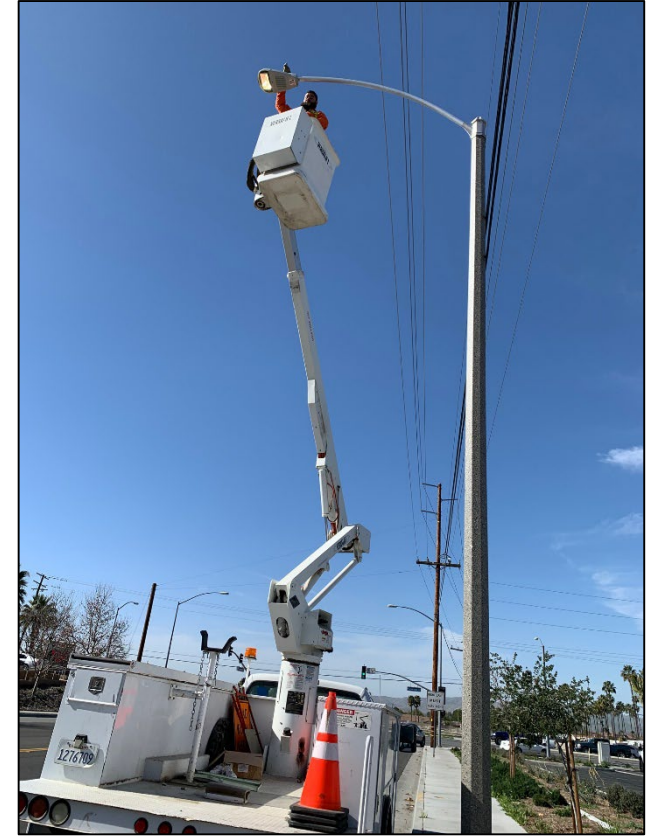
Commonwealth @ SJ Ave. Staff verified proper install of streetlight knock-down replacements
