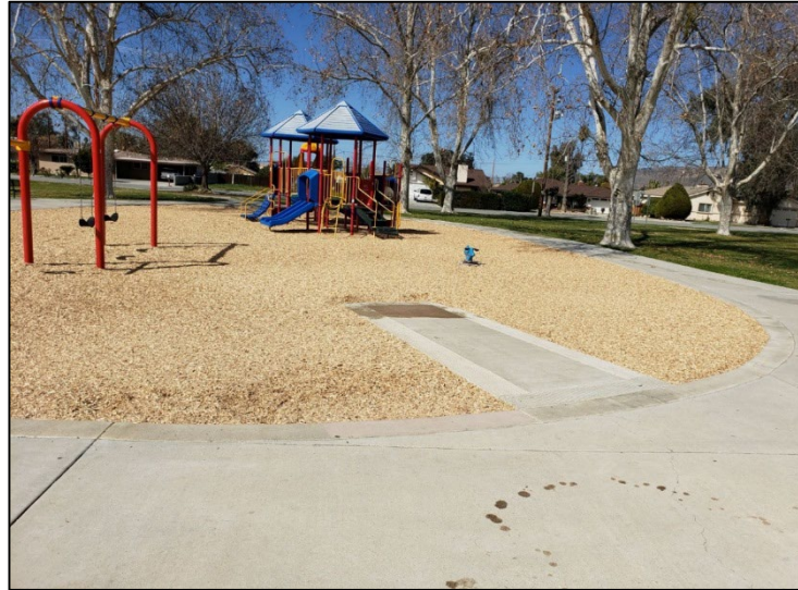
Installed 80Yds of ADA certified playground mulch at Sallee Park
