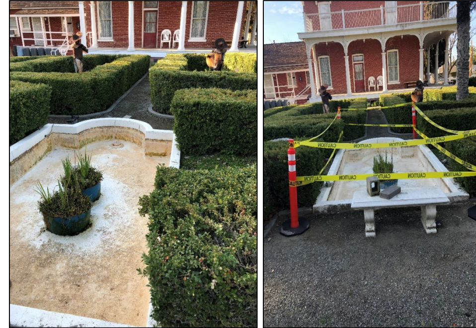
Staff drained, cleaned, & repaired cracks at the Estudillo Mansion pond
