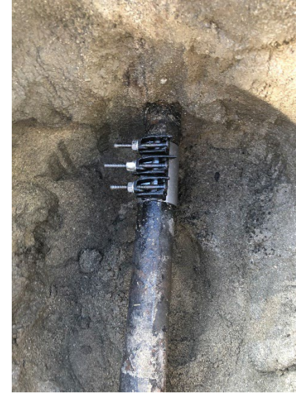
Service line leak on Mistletoe Avenue repaired
