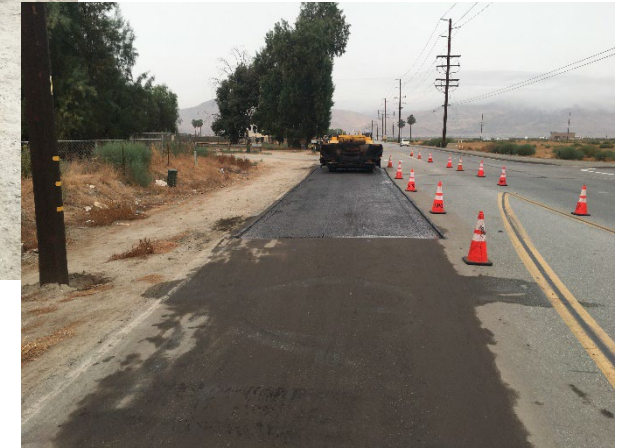
Contractor repaved sections of Cottonwood Ave at San Remo Ave
