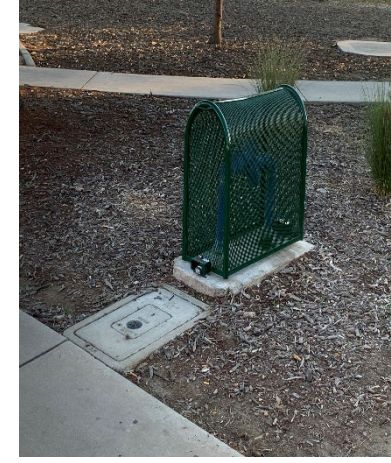
Repaired backflow and installed safety cage at Mistletoe Park
