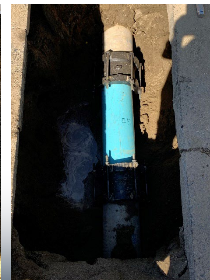
Main line leak on Hewitt Street repaired
