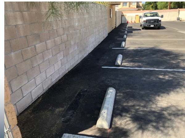
Relocated wheel stops away from the building and wall at the Police Station
