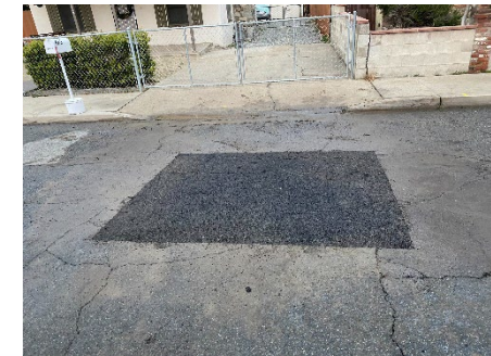
Repaired water main leak on 5 th Street
