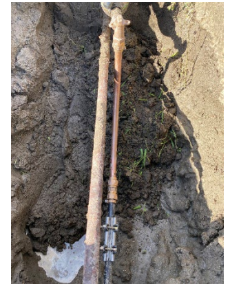
Completed service line repair on Sheriff Street
