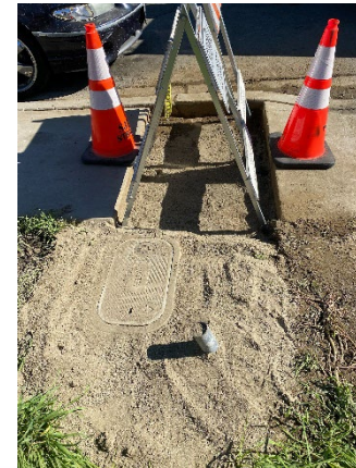
Completed service line repair on Sheriff Street
