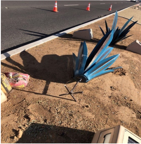
Welded additional rebar and cemented in place a replacement decorative Agave plant on the Ramona Expressway
