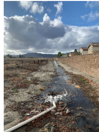
Basin de-water operations after rain events
