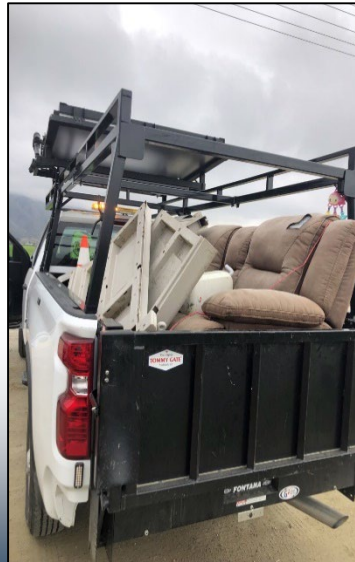
Removed illegal dumping from the right-of-way and repaired 500 square feet of potholes
