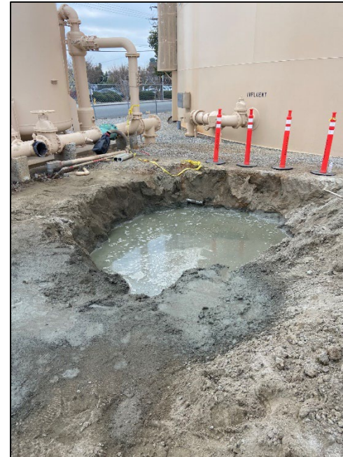
Old Grand Well Casing filled with cement slurry then inspected prior to being backfilled
