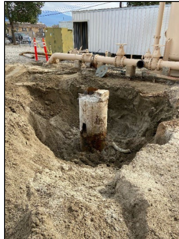
Old Grand Well Casing & Sanitary Seal exposed prior to removal
