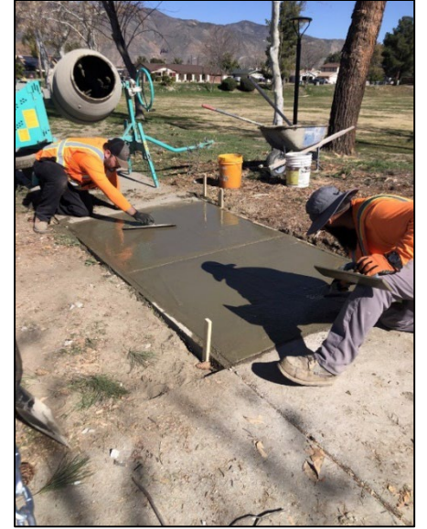
Repaired lifted sidewalk panels at various location throughout the city
