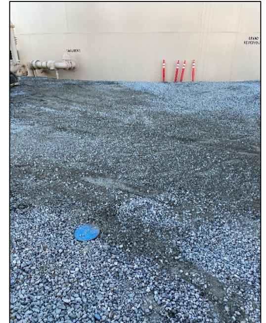
Old Grand Well Casing filled with cement slurry then inspected prior to being backfilled
