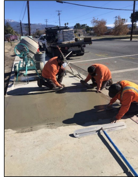
Repaired lifted sidewalk panels at various location throughout the city
