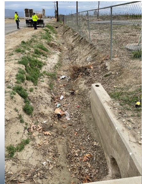
Clearing the Cottonwood Avenue Channel ▶
