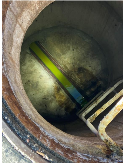
Another sewer dye test to test for sewer connection
