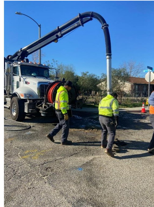
Locating a valve at Artesia and Camino Los Banos
