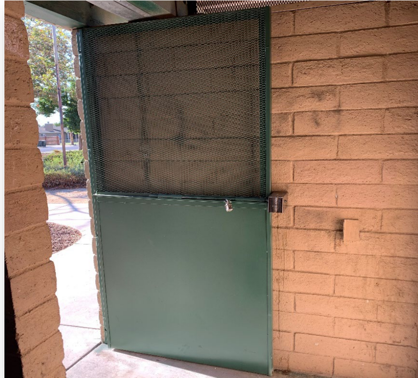
New doors installed at Mistletoe Park Restrooms
