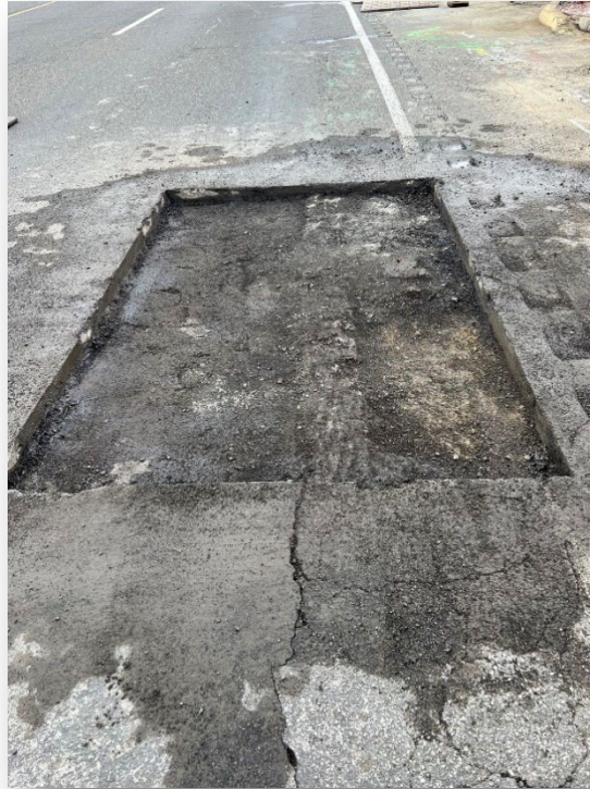
Repaired pothole on 770 N. Sanderson
