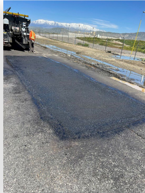
Pothole repair on 18467 Warren Road
