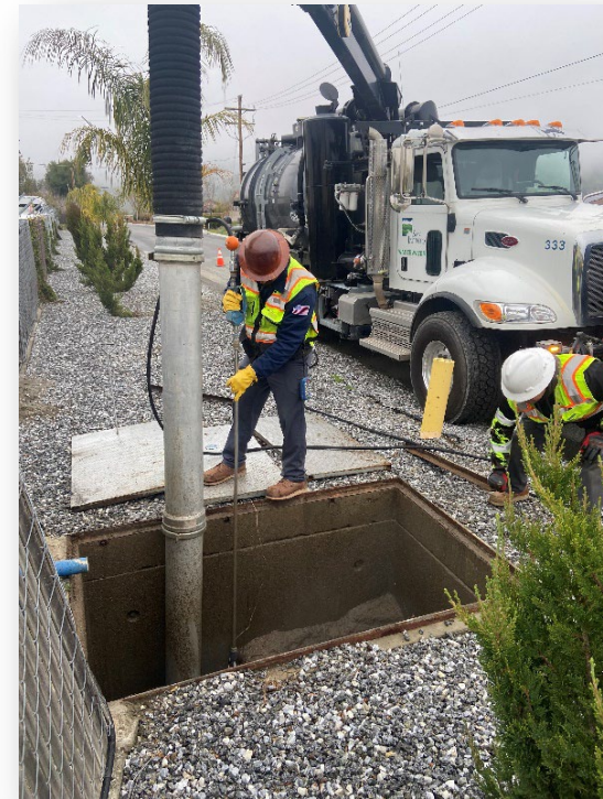
Cleaning Out a Buried Meter Vault & Preparing Meter Replacement
