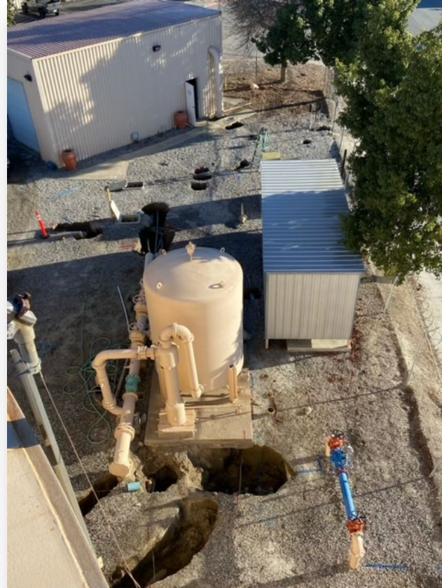
Potholing and utility location for the Grand Treatment Plan design
