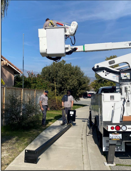
Installation of new Solar Pilot Project streetlight at Mondavi Street
