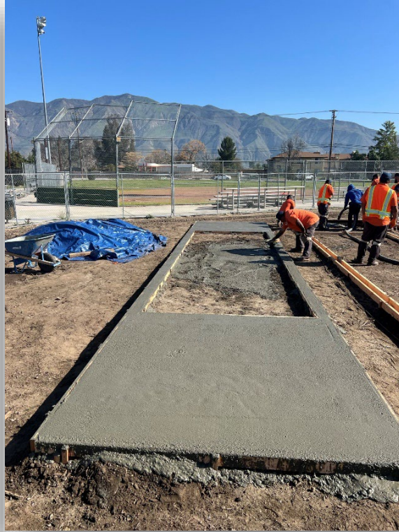
Installation of mow curbs and corn hole lanes at Sallee Park
