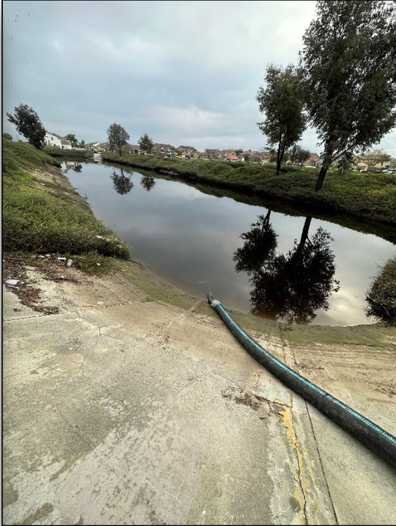
Usage of 6' tow pump to drain basis during the storm events
