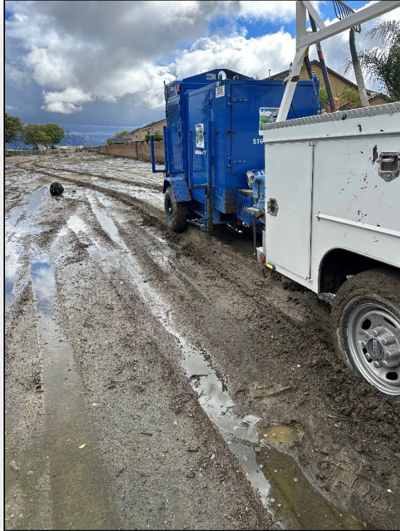
Usage of 6' tow pump to drain basis during the storm events
