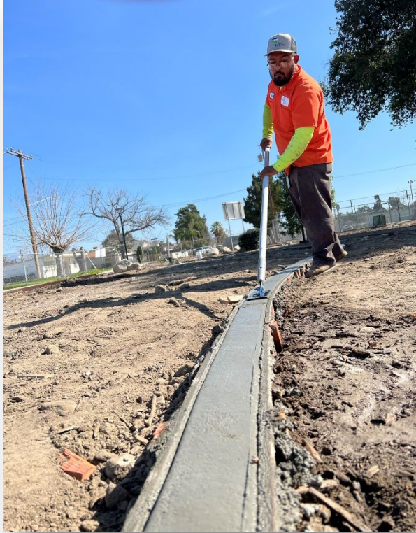
Installation of mow curbs and corn hole lanes at Sallee Park
