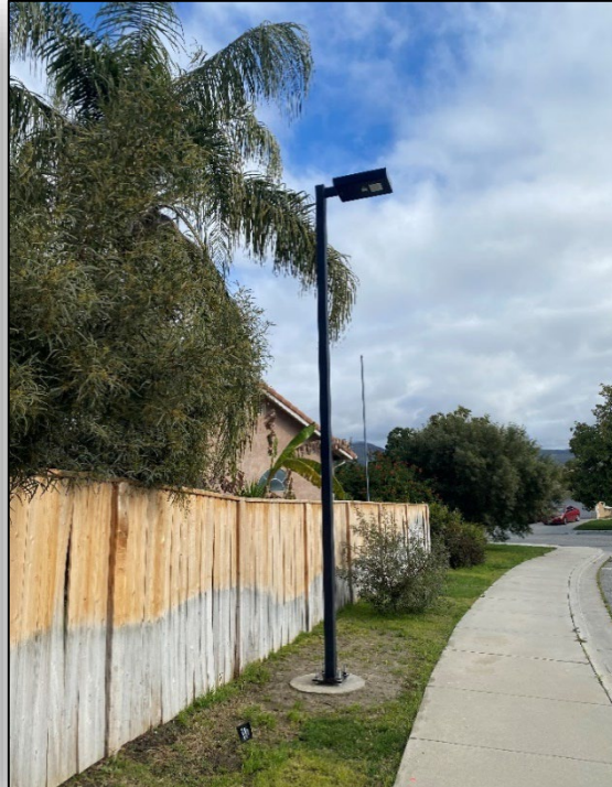
Installation of new Solar Pilot Project streetlight at Mondavi Street
