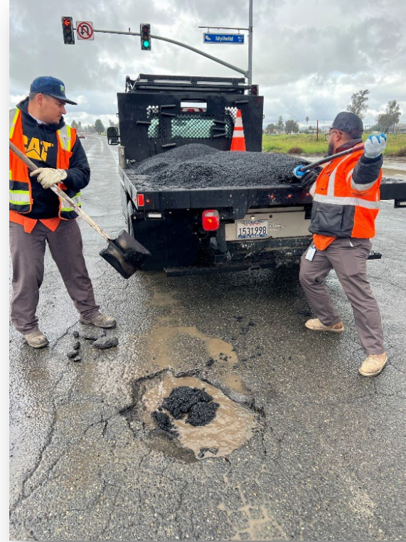
Pothole repair at Idyllwild and State
